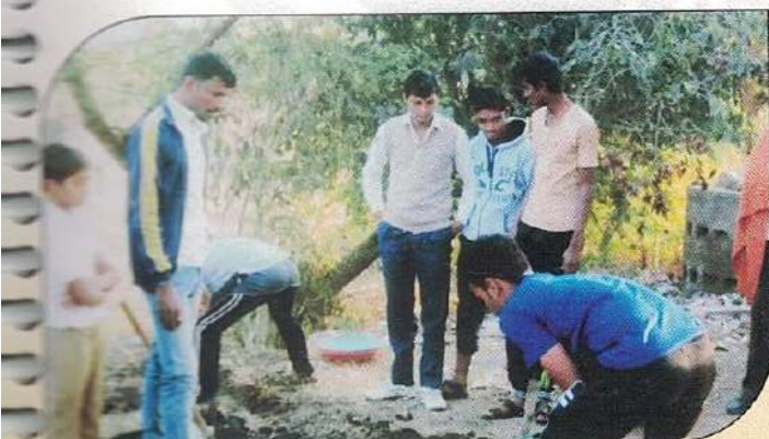
Repairing of Road
