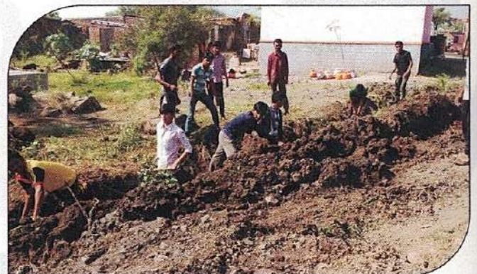
Making Ditch For Used Water
