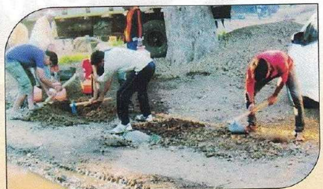
Repairing of Road
