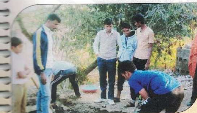
Repairing of Road
