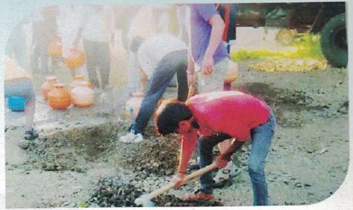
Repairing of Road
