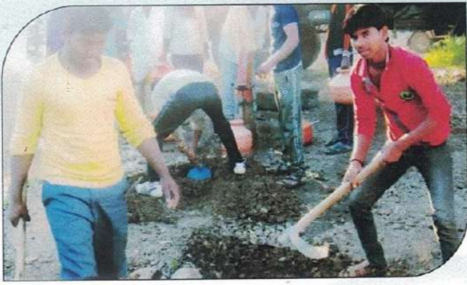
Repairing of Road
