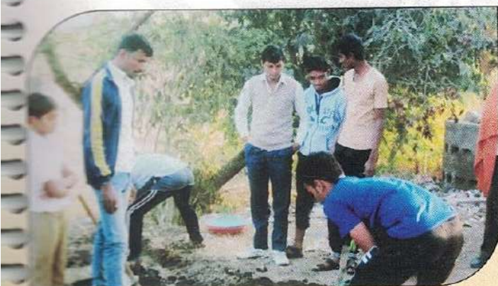
Repairing of Road
