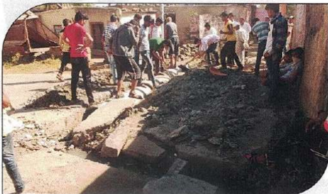
Repairing of Road
