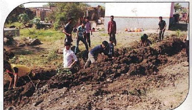
Making Ditch For Used Water
