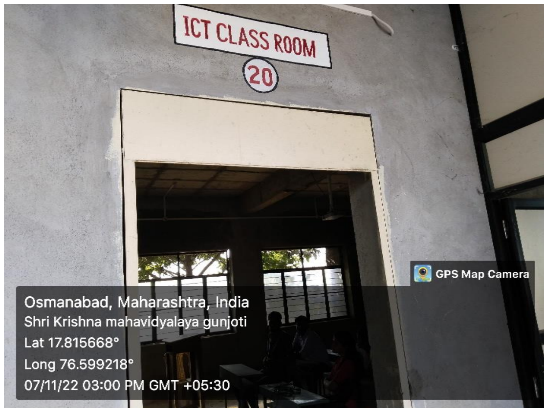
External View Of ICT Classroom No.20
