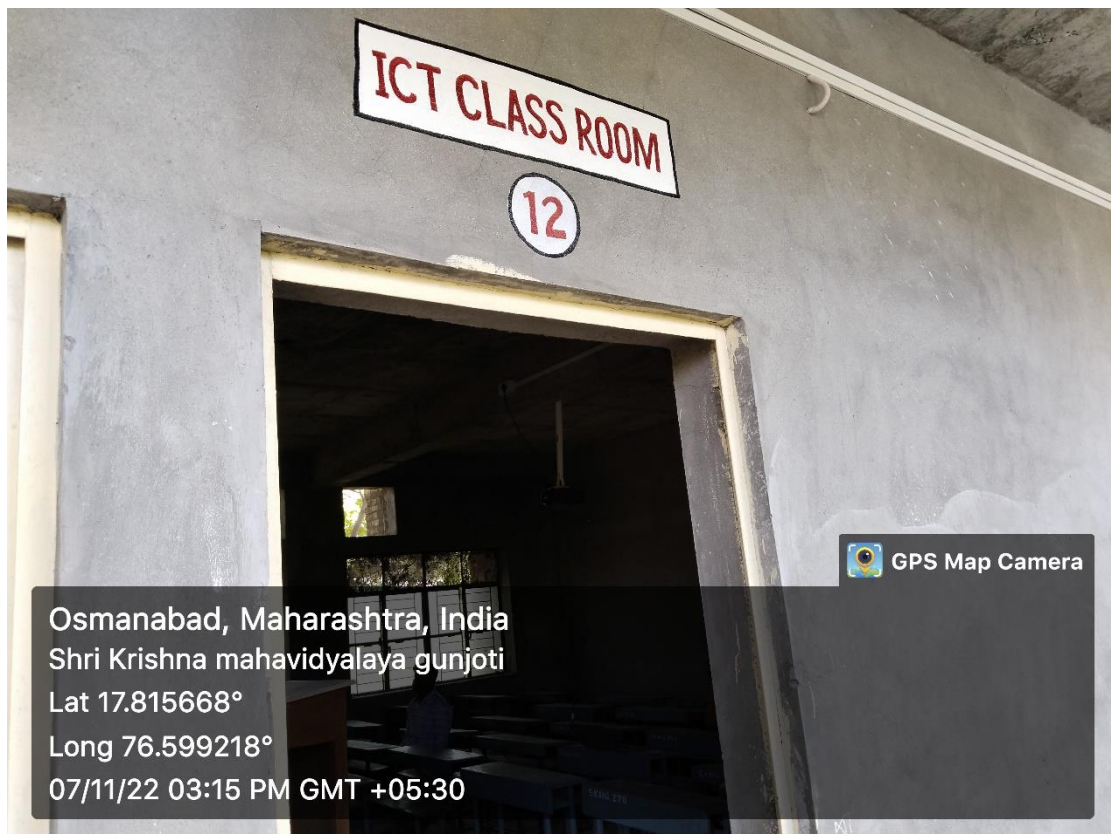
External View Of ICT Classroom No.12
